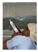
designed to be applied to the metal substrates of a roof. It adheres to aluminum, steel, and copper. Its wide range of UVresistant colours adapt to any and all decorative metal roofs and cladding products.
